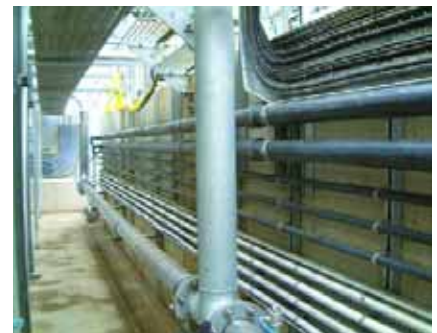
DuoSafe FLEX can easily be run in cable trays
