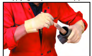
Brush applying cement to the fitting
