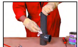
Wiping away excess cement
