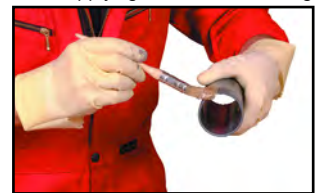
Brush applying cement to the pipe
