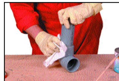
Wiping away excess cement
