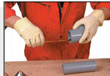
Measuring the insertion depth
