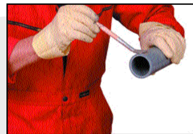
Brush applying cement to the pipe
