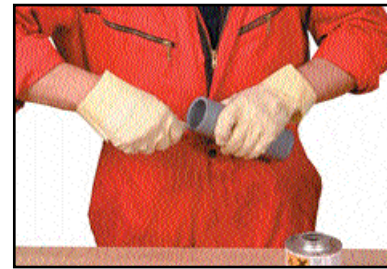
Removing the internal burr
