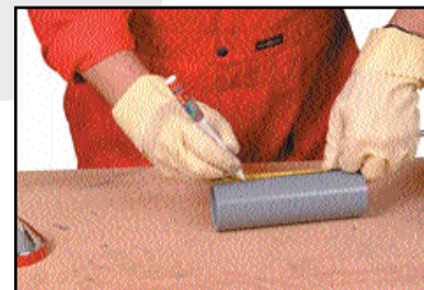
Marking the pipe end
