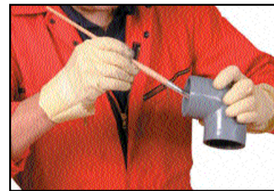
Brush applying cement to the fitting
